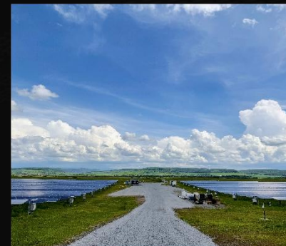
Romania Utility-scale 60MW
