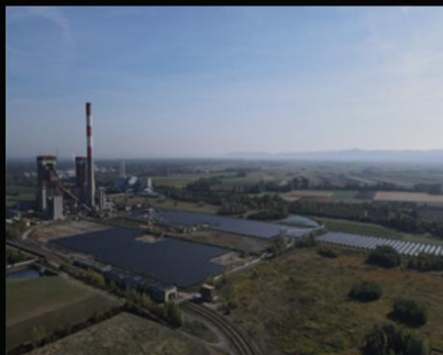
Austria Utility-scale 30.64MW
