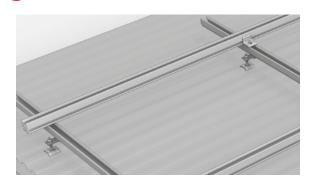
The top rail position in cross bracing is mounted with the M K2 and Climber in the desired location at the appropriate distance.
